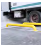
DOCK WHEEL GUIDES
